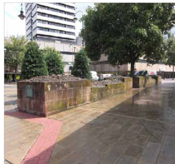
Wall remains at Spon Street
