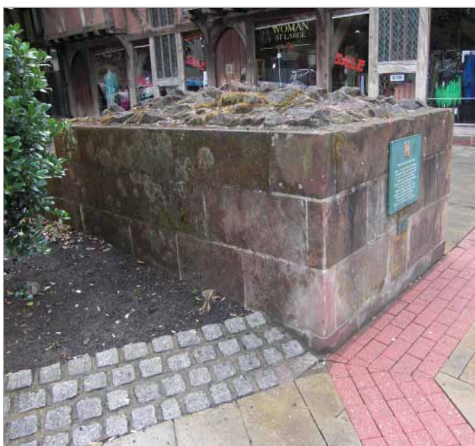
Wall remains at Spon Street
