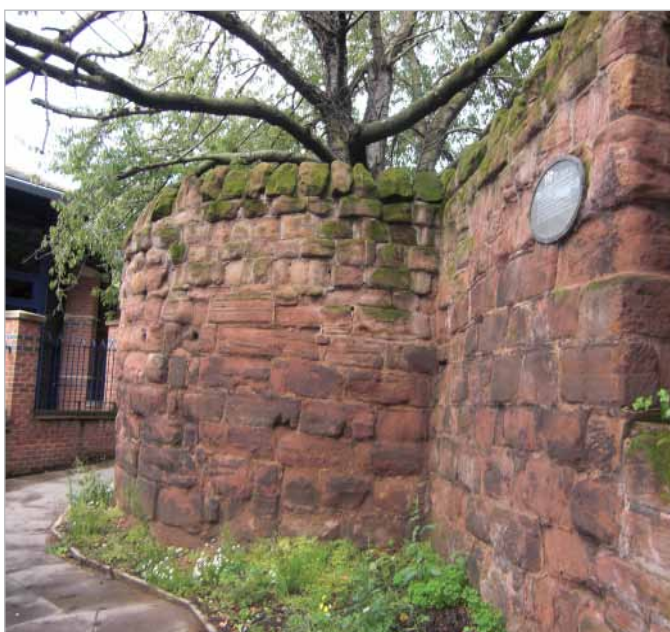
Wall and Bastion near Well Street
