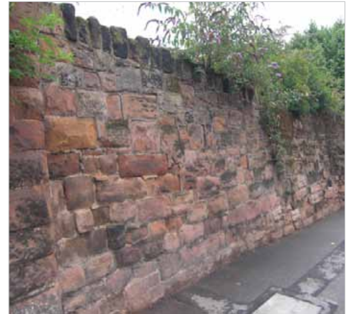
Wall at Gulson Road
